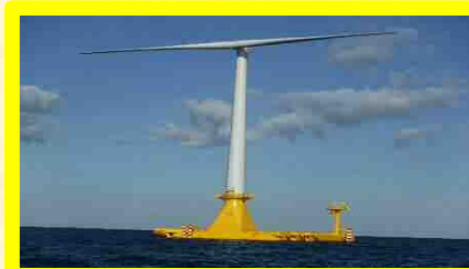
Japan's First Barge-type Floating Offshore Wind Farm Demonstration
